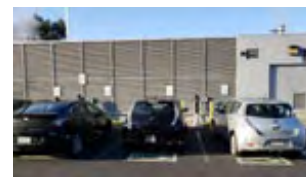
Charging station (United States)
