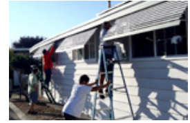
House rehabilitation activities
