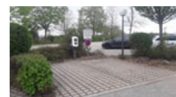
Charging station (Germany)
